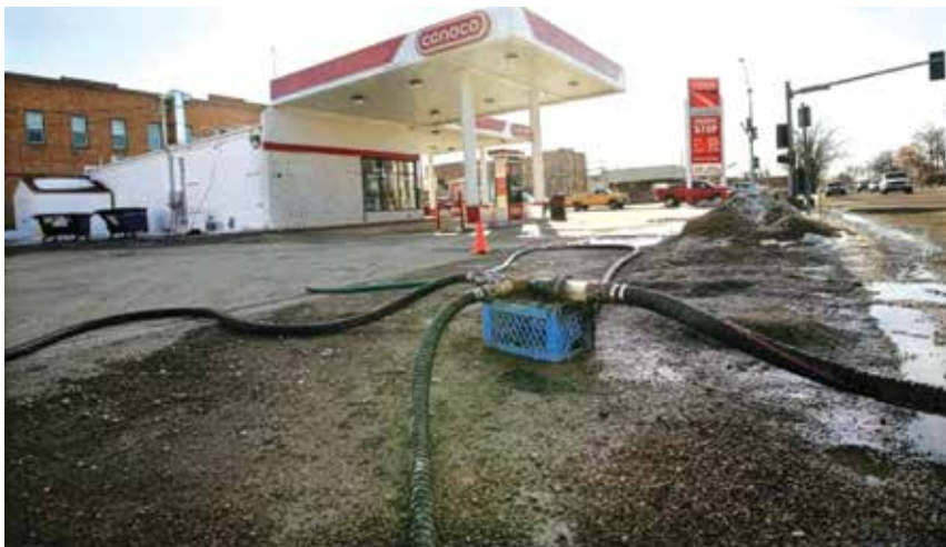
Gas station cleanup from Billings Gazette
